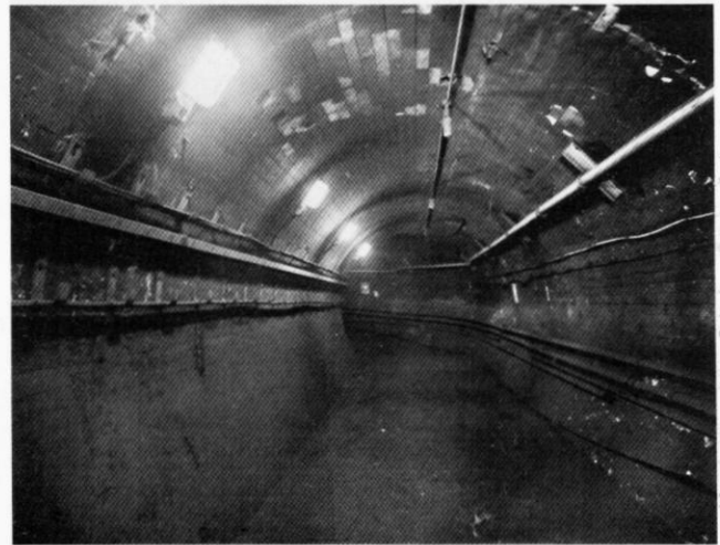
Subway from lower lift landing to the City Road southbound platform. Photo Nick Catford
